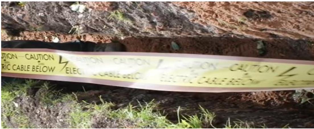
Figure 2: Cable and duct warning
